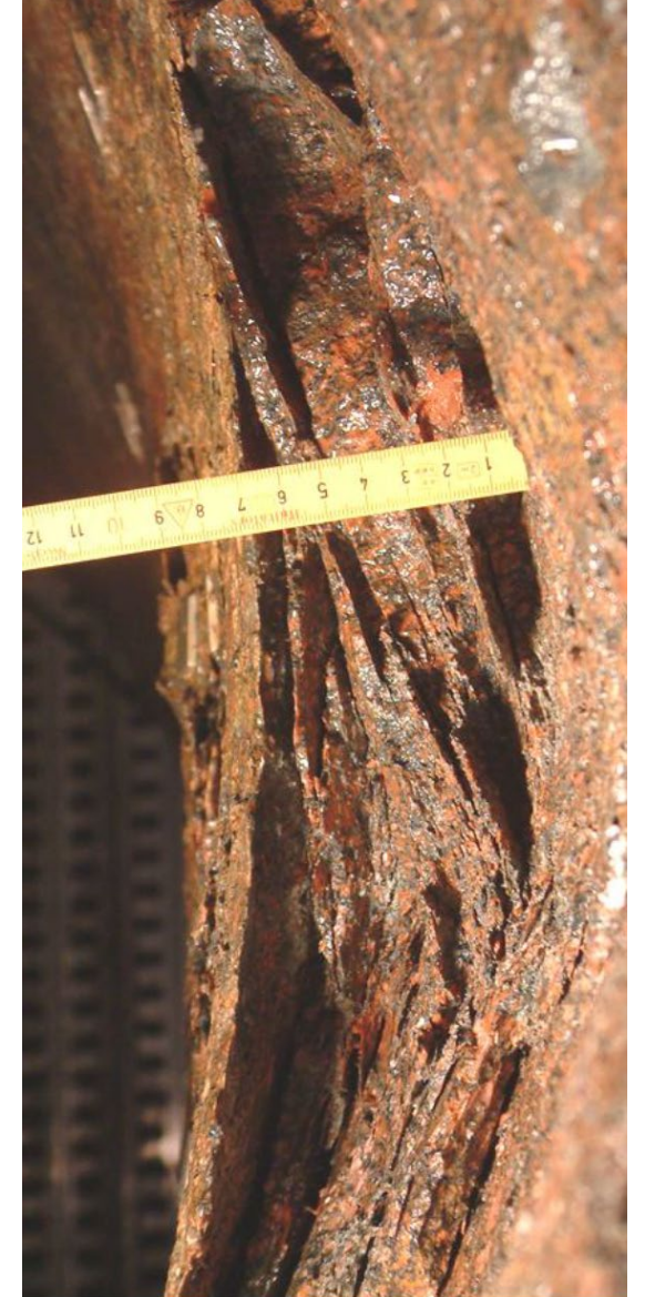
thin slabs, buckled
