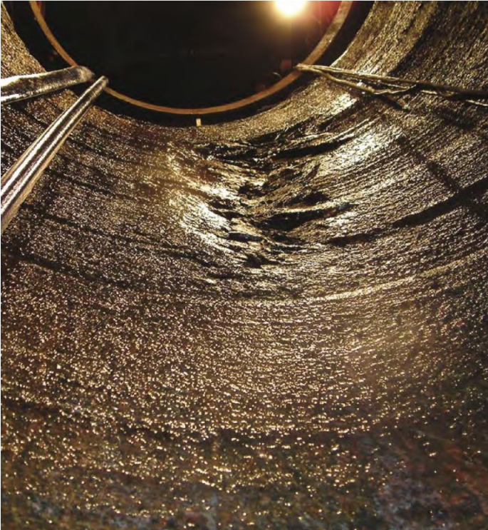
Initial spalling during drilling
